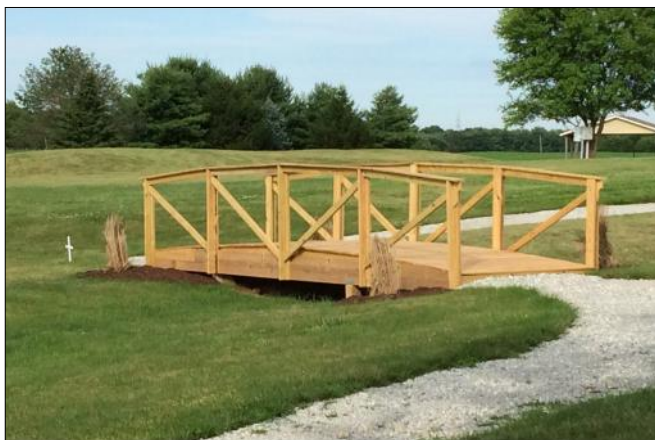
Finished bridge financed by youth grant.
